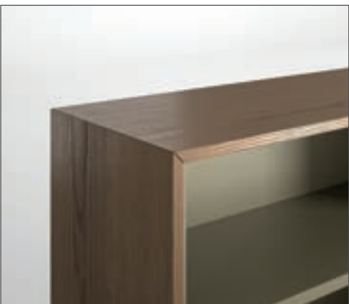
Miter joint 20 Inglete 20mm *Detail/ Detalle p.128
